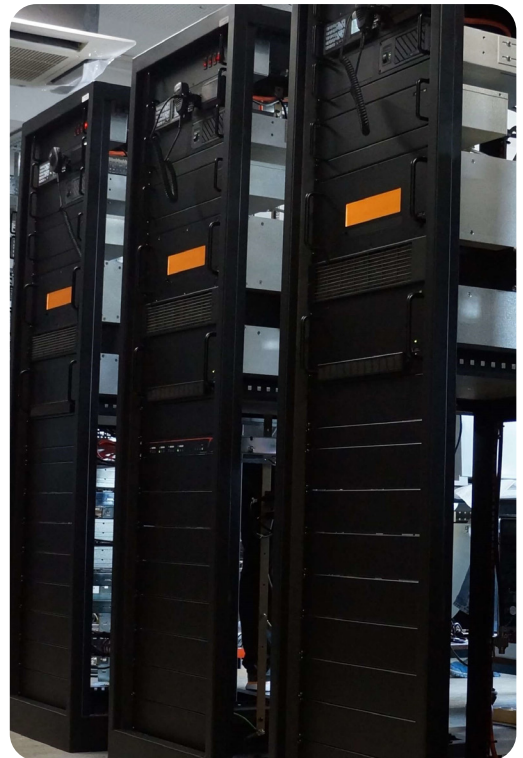
Multiple-racks for large scale systems.
